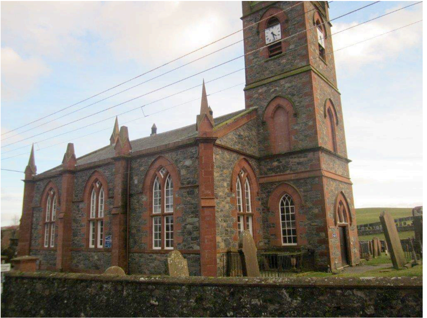
North elevation to Kirkgate
